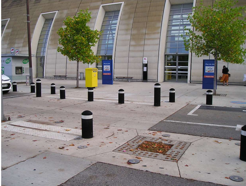
Figure 65: Example of bollards that could be used to separate the carriageway from the pedestrian walkway
